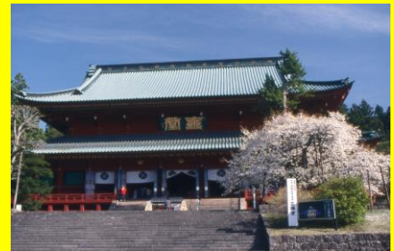
Rinnoji Temple (Under renovation)
